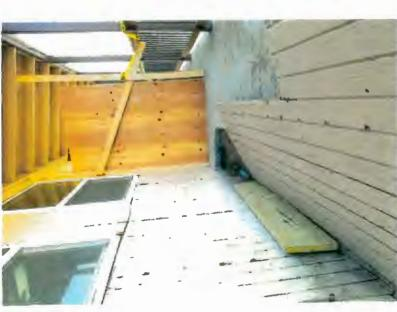
Facilities Maintenance discovered termite damage, blocked off the area, and recommended our program hire a Contractor for repair work.
