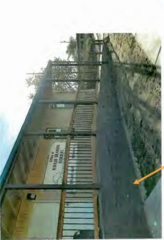
Based on Navajo Nation Facilities Maintenance Department's assessment, this cinder block wall needs to be torn down and rebuilt.
