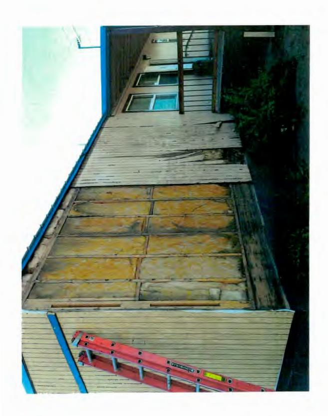
Termite damage to the floor joist and wall membrane near the front entrance area.
