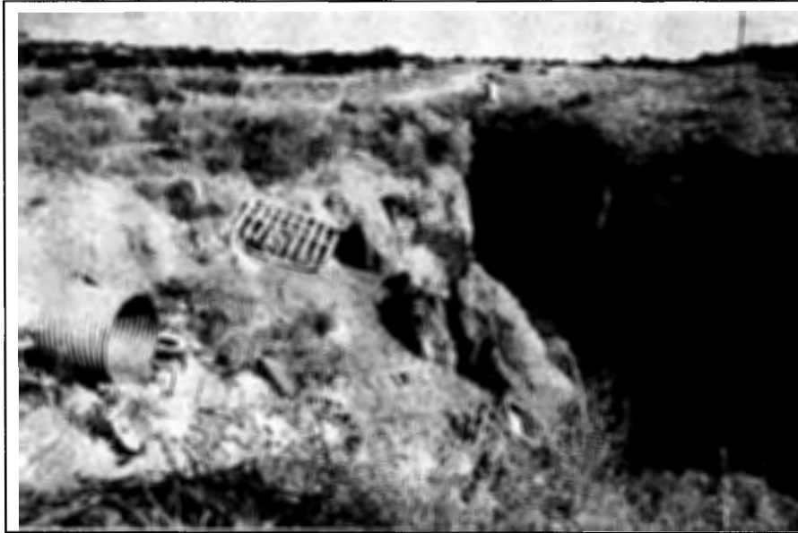
19. Heavily eroded culvert crossing east of Borrego Pass
