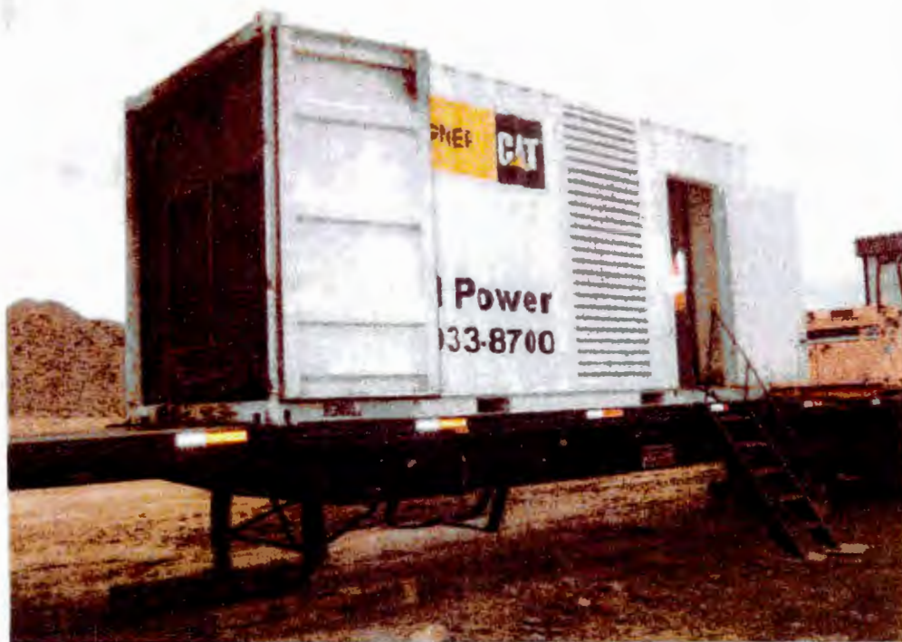
Photograph 8: View of Unit 17-115 CAT 725 KW diesel generator. Diesel tank is housed inside generator to the right of the doorway.
