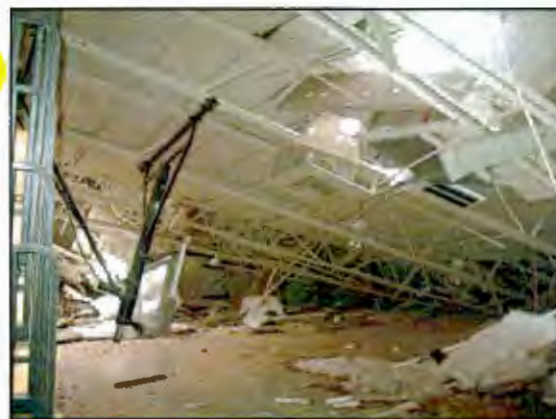
The gym roof collapsed in January at Shonto Preparatory School in Arizona. The gym was built in 1966.
