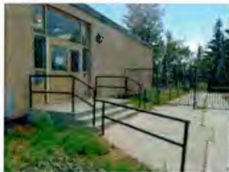
Lack of ramp accessibility wings A and B
