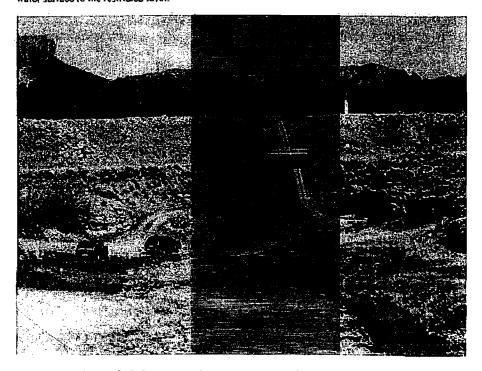
Figure 5. View of siphons on downstream embankment of Tsaile Dam. Siphons were discharging 22 cfs (April 2005).
