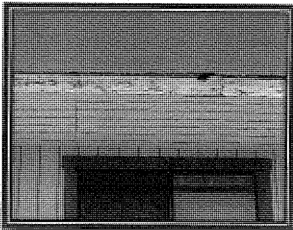
Photo 32: Flaking paint, suspect lead based.
