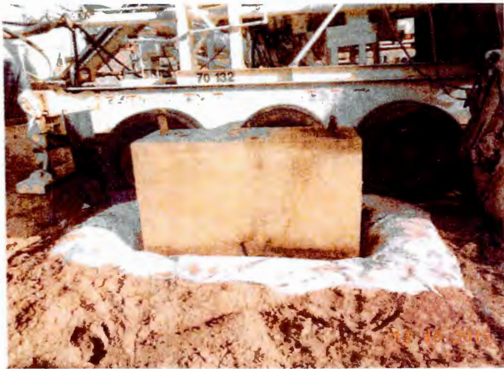
Photograph 1: View of 200-gallon diesel fuel tank for No. 2 diesel fuel use.
