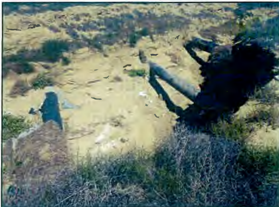
Photo 8. Three of the four pipelines in a wash, exposed by erosion.
