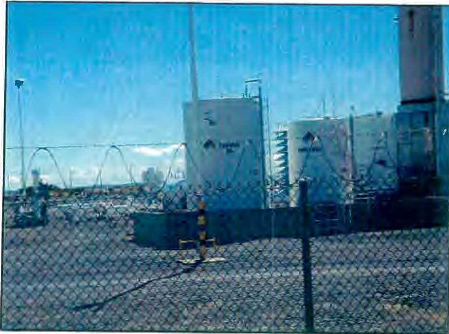
Photo 17. Three large ASTs in secondary containment were in the main part of the compressor station. They were labeled turbine oil, ambitrol, and used oil.
