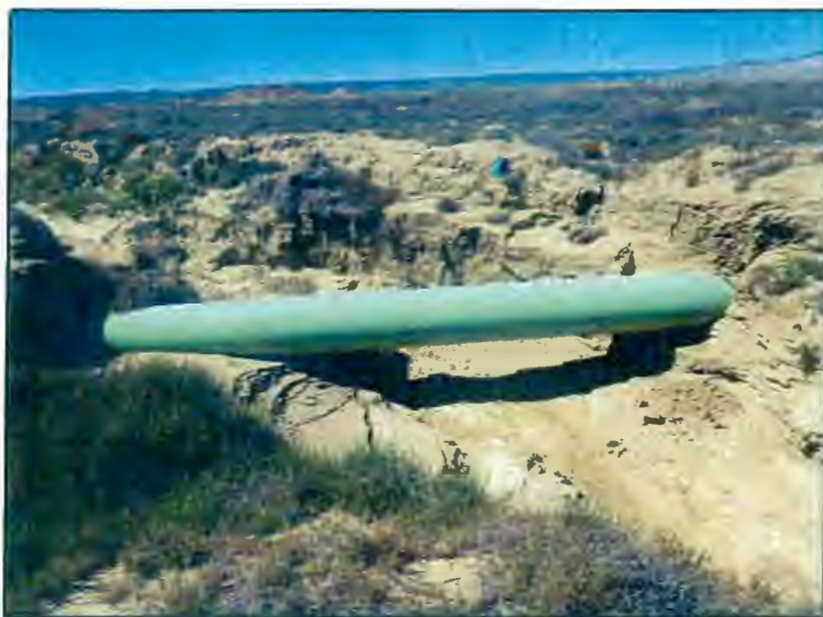
Photo 9. The fourth pipeline in the wash, exposed by erosion.
