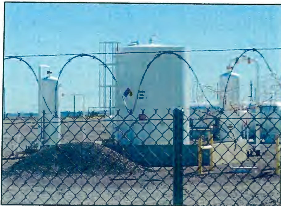
Photo 18. This is the used oil AST at the main part of the compressor station.
