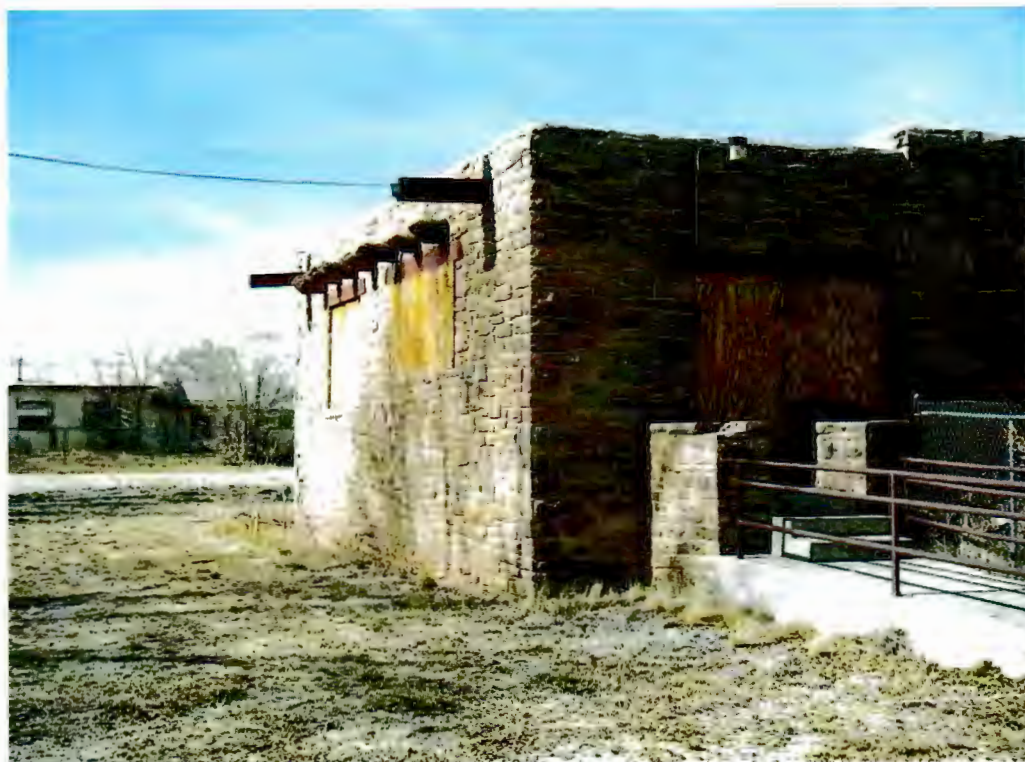
Photograph 3. Building 901 showing stone masonry and vigas.
