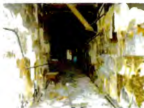
Fire damage to South end hall stucco wall.
