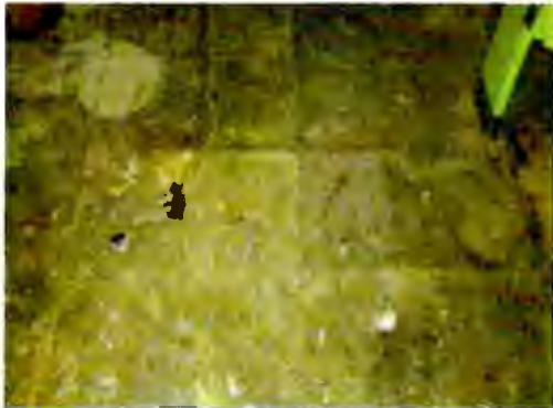
North restroom floor tiles. 10% Chrysotile
