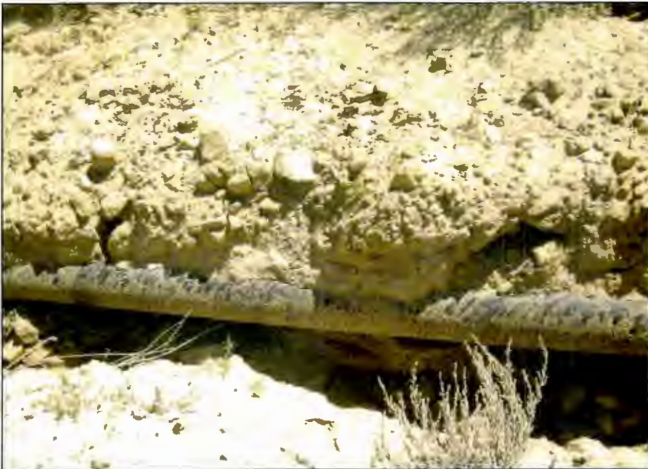
Existing Pipeline: Existing pipeline corridor, exposed pipeline
