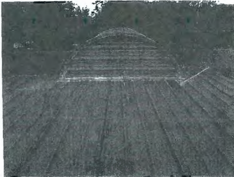
The "dome" above the front entrance, note the visible sign of dirt and moisture at the edge of dome. Should have some slope to have water run off to drainage. Presently water drains in wall cavity of men's restroom.
