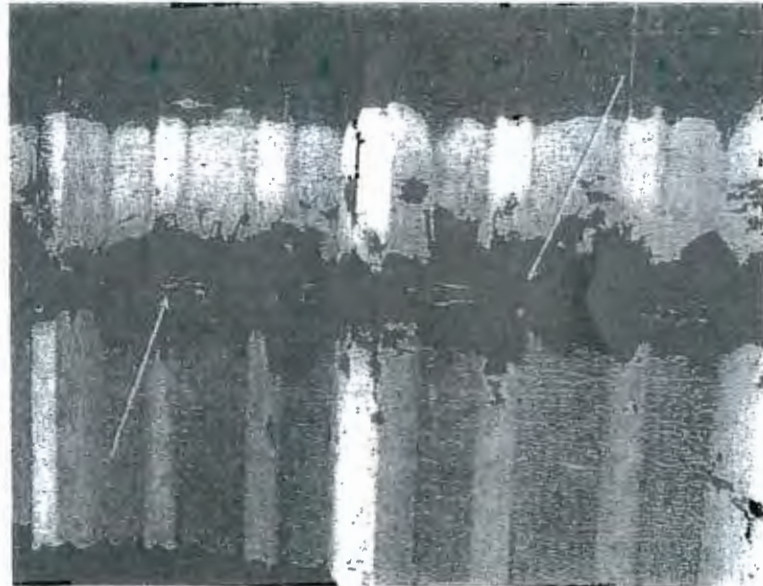
Close of weather and damage sealants at seams of pro-metal panels. It is suspected that the screws have buckle from the expansion and contraction of materials.
