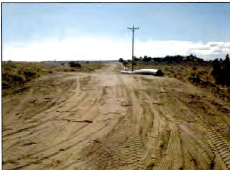
Long view of typical 100-foot disturbance right-of-way for the NGWSP; installation for 22-inch or greater diameter HDPE pipe. Photo not from Reach 26.3, which would install 12-inch diameter or less pipe.
