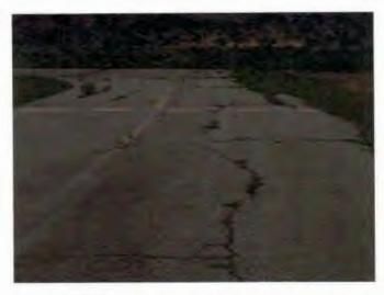
Taxiway to Runway 20 exhibits cracking with vegetation growing into the cracks.
