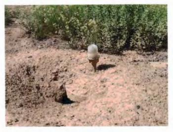
Runway lights are stake-mounted and vulnerable to rodent damage.
