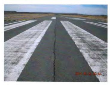
A closer look at Runway 15 end looking south. Here is an example of longitudinal pavement cracking prevalent down the runway short of 1500 feet from south end.
