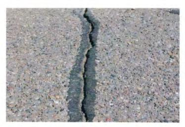
Runway cracks have been cracksealed in past years, but continue to widen requiring additional crack-seal or repair.
