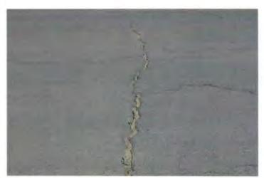
Example of a lateral crack in the runway filled with dirt and some vegetation.
