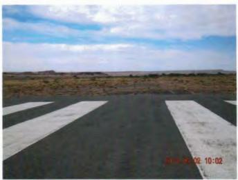
From the threshold of Runway 33 looking south; Markings are faded, however pavement appears to be in better condition than the north end.
