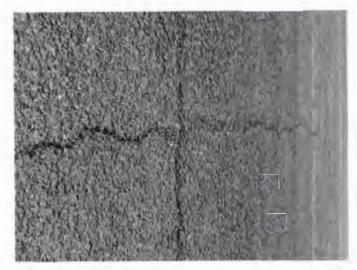
Typical cracking patterns throughout the length of the runway are apparent.
