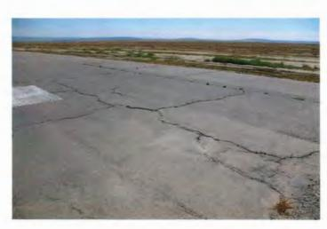
A closer look at Runway 2 end shows an example of longitudinal pavement cracking prevalent down the runway.
