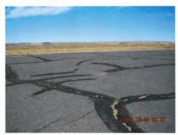
Wide block cracking with old crack seal; vegetation is growing through the cracks.
