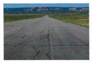
Approach end of Runway 18 looking south; Example of longitudinal cracking in foreground; A large dip in the runway occurs at mid-field.
