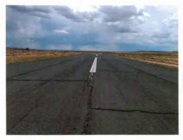
Extensive cracking throughout the runway surfaces, most with vegetation established inside of the cracks.
