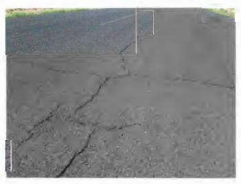
Cracking and possible pavement failure issues at mid-field on Runway 02/20.
