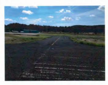
Taxiway tie-in to Runway 20; Pavement is in fair condition; markings are very poor and faded.
