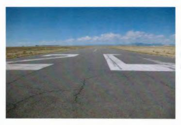
Runway 20 approach looking down the runway; pavement cracking is evident and is in need of crack-sealing.
