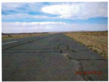
Looking north from mid-field; Vegetation has begun to work its way into the open cracks.
