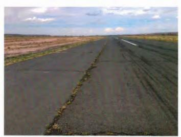
Longitudinal cracking full length of the runway
