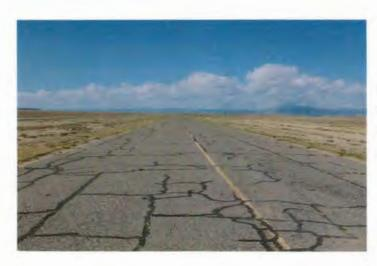
Partial-parallel taxiway with widespread cracking; pavement is fair condition, with previous crack seal applications evident.
