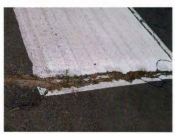
Close up of marking and asphalt cracking and vegetation on north end of the runway.
