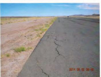
West side of the runway at mid-field; A section of the shoulder has begun to crack and fail.
