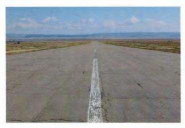
Centerline markings are faded and in poor condition.
