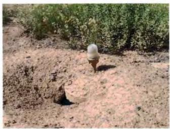
Runway lights are stake-mounted and vulnerable to rodent damage.
