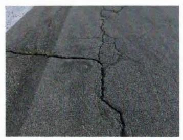
Example of cracking and potential asphalt failure near mid-field.
