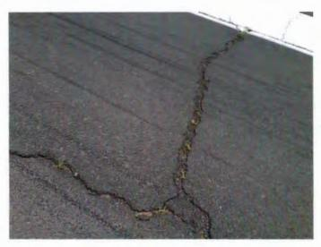
Lateral cracking with vegetation beginning to work its way into most of the cracks.
