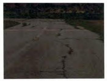
Taxiway to Runway 20 exhibits cracking with vegetation growing into the cracks.
