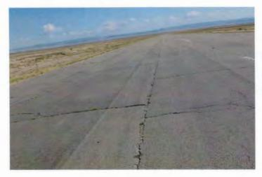
Example of both longitudinal and lateral cracking present throughout the runway.
