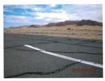
Approximately 1,500 feet south of the approach end of Runway 15, a large section of cracked, rough, and heaved pavement is present; it is possibly the result of expansive soils in the pavement sub-grade.
