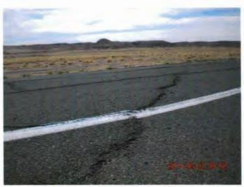
Major cracking and associated heaving is occurring transversely across the runway.
