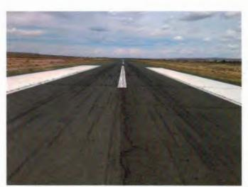
A closer look at Runway 18 end looking north. Here is an example of longitudinal pavement cracking prevalent down the runway short of 1500 feet from south end.
