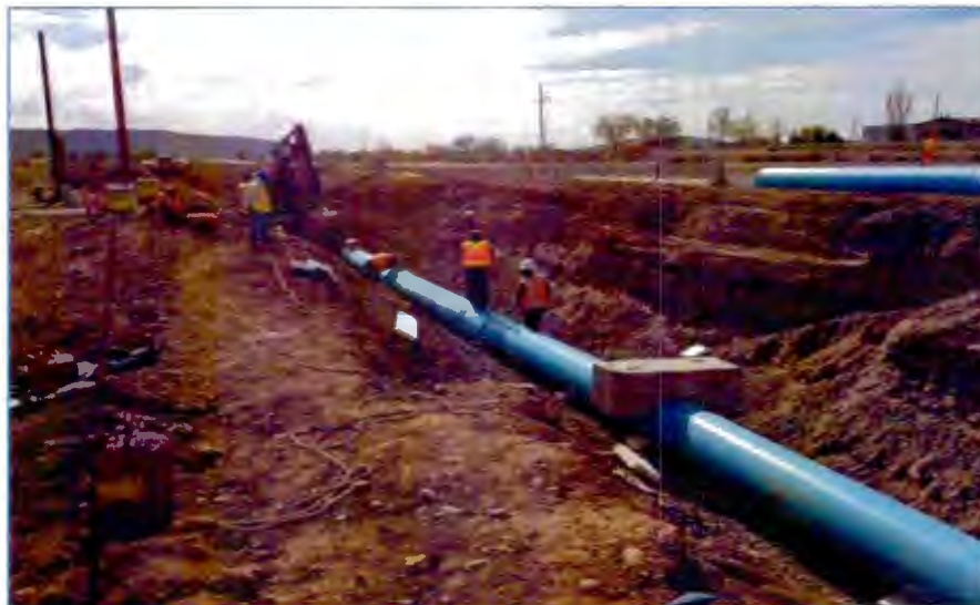
Figure 7. Typical trench and pipeline construction adjacent to public roads
