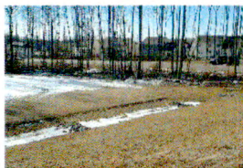
Check dams are used to reduce the energy of stormwater to prevent erosion
